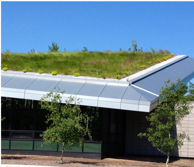
ABOVE:| Innisfail Library
