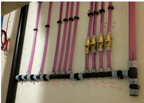
TOP LEFT: Modular cisterns are available for different surface-weight loadings. To be used as a cistern, they are wrapped in a waterproof membrane, using the same technology and installers as are used for basement radon-proofing. TOP RIGHT: Cartridge filter canisters below (blue) and UV disinfection above. BOTTOM: Purple-pipe distribution manifold in a home with rainwater used for toilet flushing.
